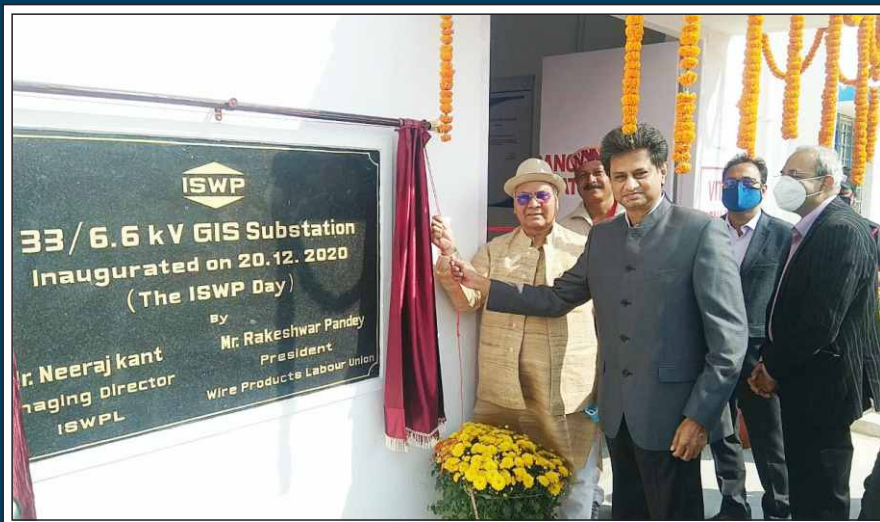
Inauguration of 33 kV GIS Substation at ISWP by Mr. Neeraj Kant, MD ISWP & Mr. Rakeshwar Pandey, President, Wire Products Labour Union
